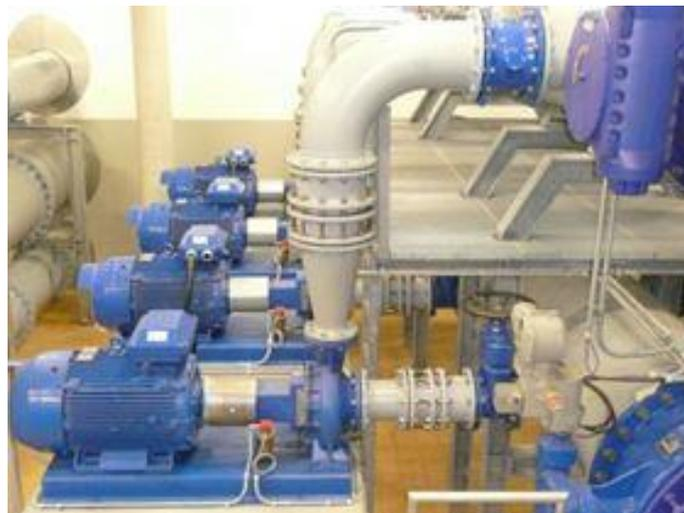
Fig.2.15 PAT installation in the pumping station at Breech, Germany [26]
