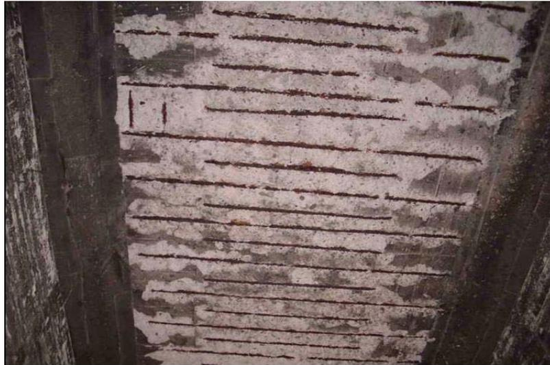
(a) Corrosion of reinforcement in a bridge deck slab
