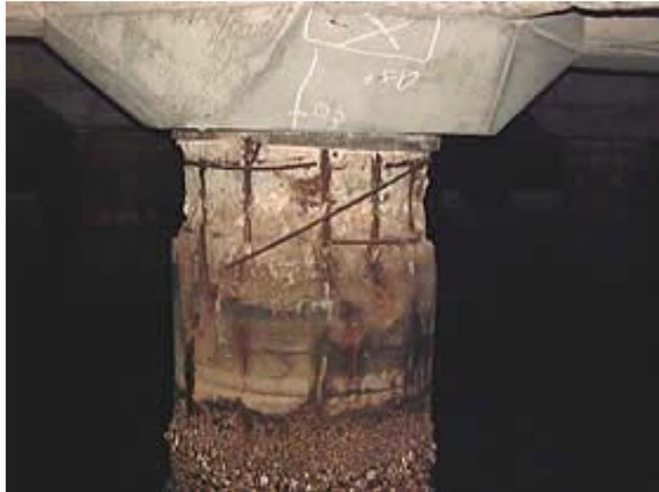
(c) Corrosion of reinforcement in a bridge pier
