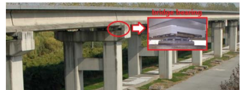
(e) Bridge bearings between the girder and pier
