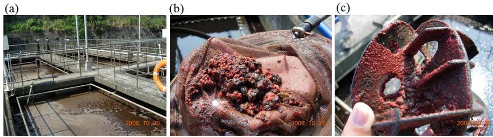
Fig. 2-4 The full-scale anammox reactor in Taiwan treating landfill leachate (a) Aeration tank; (b) suspended anammox biomass; (c) attached anammox biomass (Wang et al. 2010).
