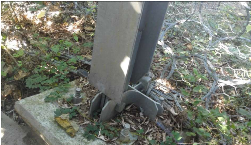
Figure 2-7. Photograph of the rotatable joint and the foundation of a supporting post
