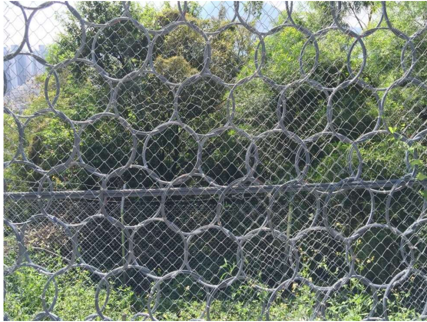
Figure 2-3. Photograph of the flexible ring net
