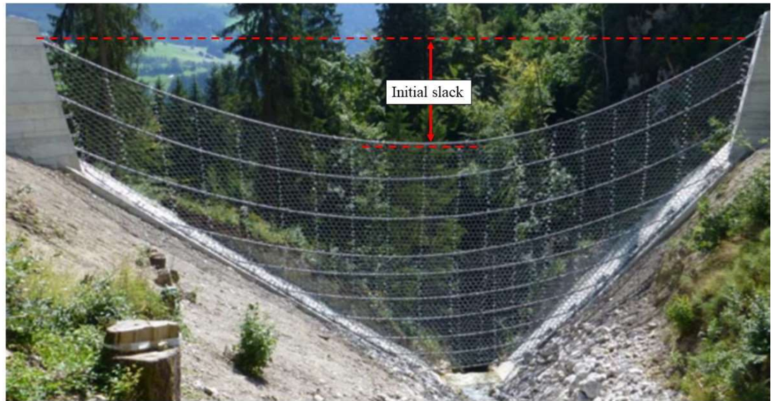
Figure 8-1. Initial slack of the supporting cables due to the self-weight of the flexible ring net (Wendeler et al. 2018)
