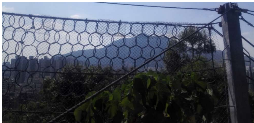
Figure 2-4. Photograph of strand cables and cross tension cables
