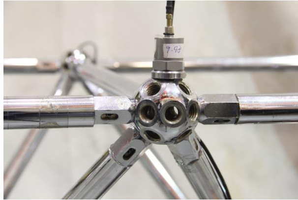
Figure 3.25 Accelerometer at the Meroform ball node
